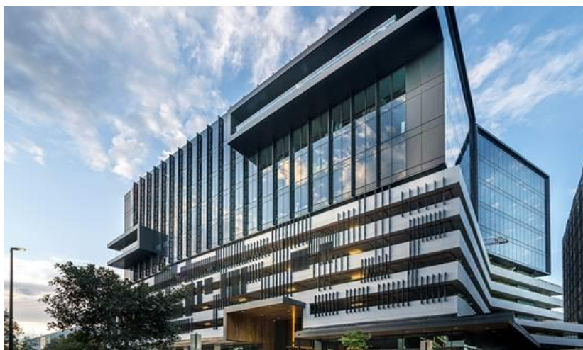
Connect Corporate Centre – Building 2
