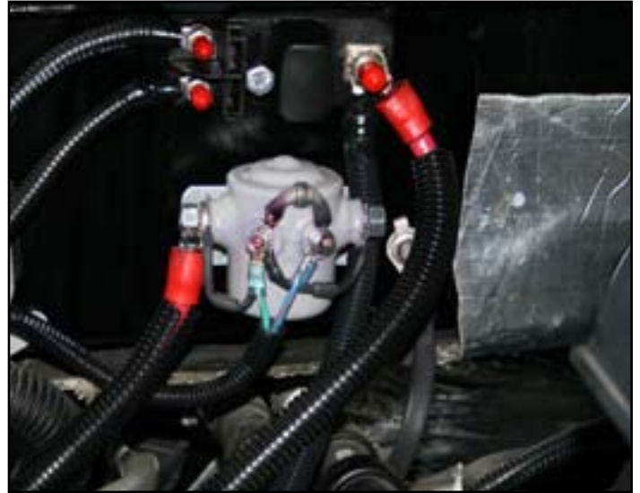
Navigator power distribution module under the hood
